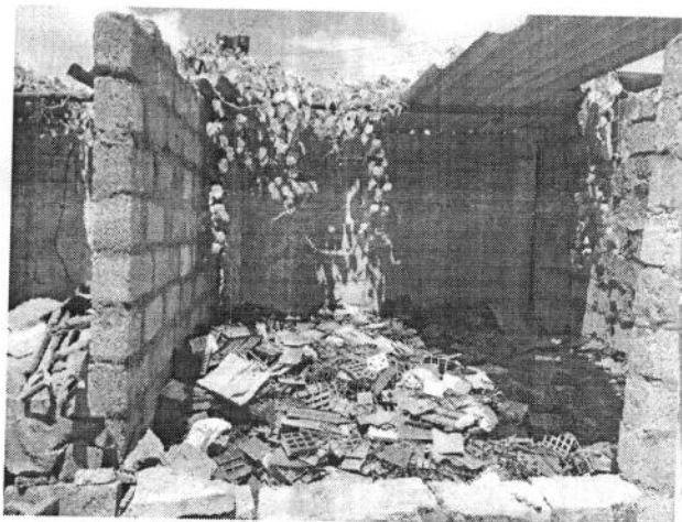
Damaged/Collapsed Roof of slag, ash & Dismantled components
