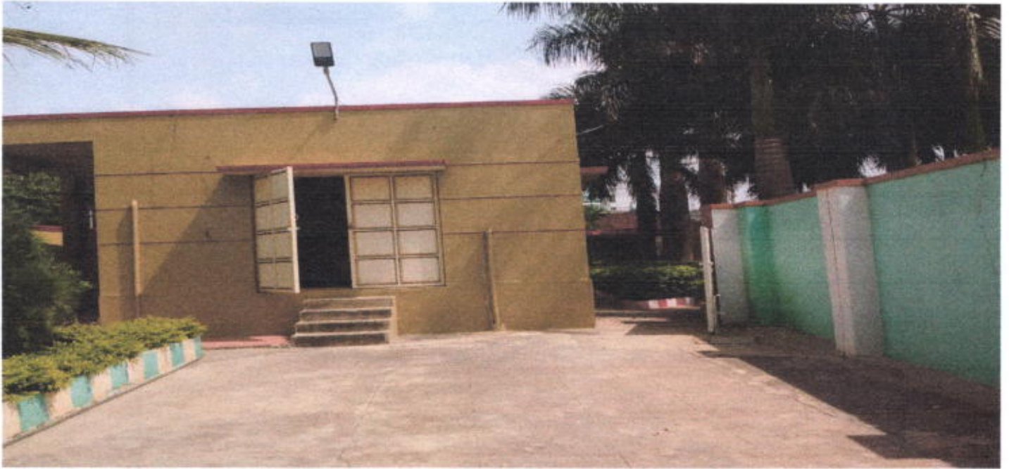
62.5 KVA DG Set provided in a closed room
