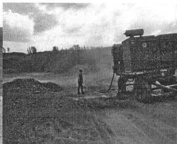
Water Canon for dust suppression
